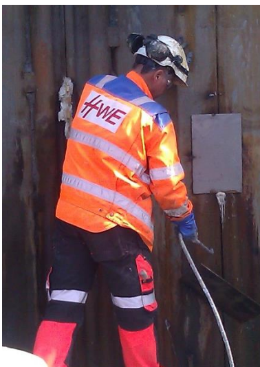
Figure 6 Sealing sheet pile interlocks and openings by grouting water reactive polyurethane HAG
