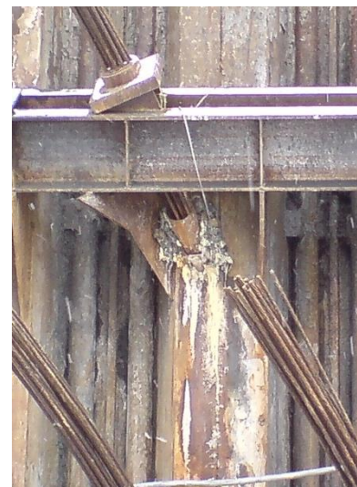
Figure 6 Sealing sheet pile interlocks and openings by grouting water reactive polyurethane HAG
