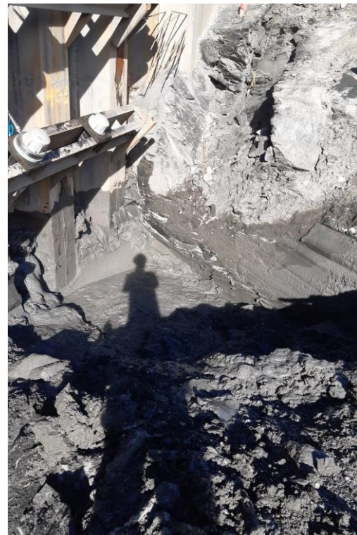
Figure 14 Polyurethane mixed with clay
