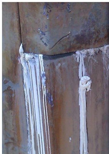
Figure 6 Sealing sheet pile interlocks and openings by grouting water reactive polyurethane HAG
